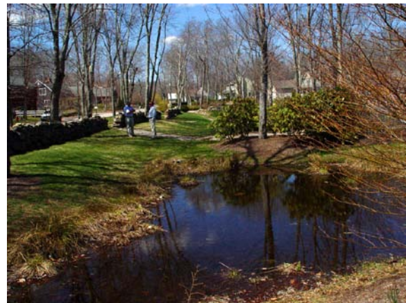
Figures 12 and 13 Infiltration meadows, promoting aquifer recharge, are a less expensive, more attractive, and environmentally superior alternative to deep “bomb-crater” basin design, and are very easy to create when lot sizes are reduced to provide common open space. In this example from Doylestown Twp., the side slopes are so gentle that the entire “facility” can be mowed with large equipment just once a year, a cost saving that also allows the area to function as wildlife habitat throughout the summer, attracting birds, bats, insects, small mammals, and raptors. Small seasonal ponds can also enhance roadside open space, such as shown here in a modest neighborhood green encircled by a residential street.
