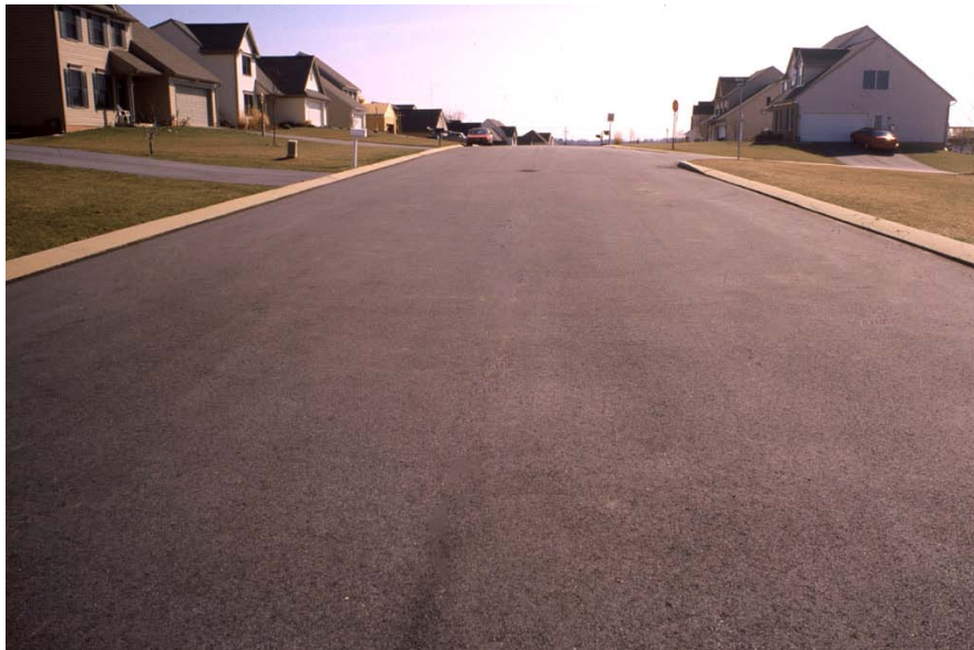
Fig. 1 What’s wrong with this picture, taken in Lancaster County, but typical across the Commonwealth? (Clue: Typical subdivision street standards that specify excessive cartway width, which leads to increased vehicular travel speed, while not even requiring sidewalks for pedestrian safety or shade trees for neighborhood beauty.)
