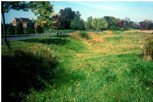
Figures 12 and 13 Infiltration meadows, promoting aquifer recharge, are a less expensive, more attractive, and environmentally superior alternative to deep “bomb-crater” basin design, and are very easy to create when lot sizes are reduced to provide common open space. In this example from Doylestown Twp., the side slopes are so gentle that the entire “facility” can be mowed with large equipment just once a year, a cost saving that also allows the area to function as wildlife habitat throughout the summer, attracting birds, bats, insects, small mammals, and raptors. Small seasonal ponds can also enhance roadside open space, such as shown here in a modest neighborhood green encircled by a residential street.
