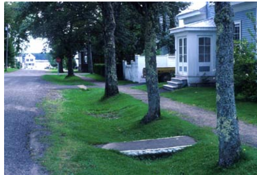
Fig. 11 Swales can easily serve in place of curbs, even when density is more than two or three dwellings per acre.
